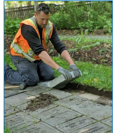
Installing memorial pavers.
