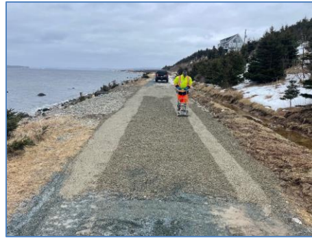
T'Railway Repairs, CBS
